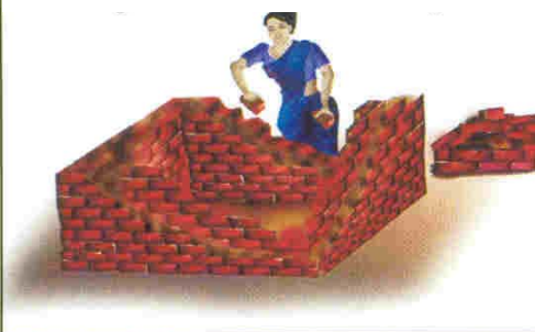
2. Erecting double wall with cavity
