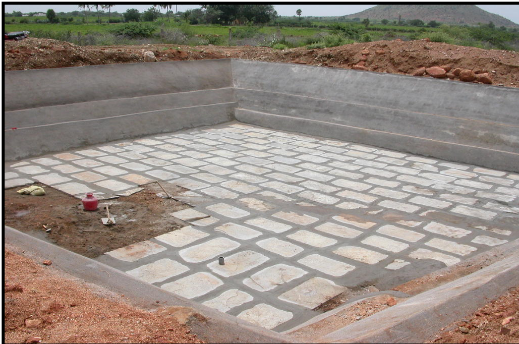
Fig. 15.4 Farm Pond Lined with Fire Bricks
