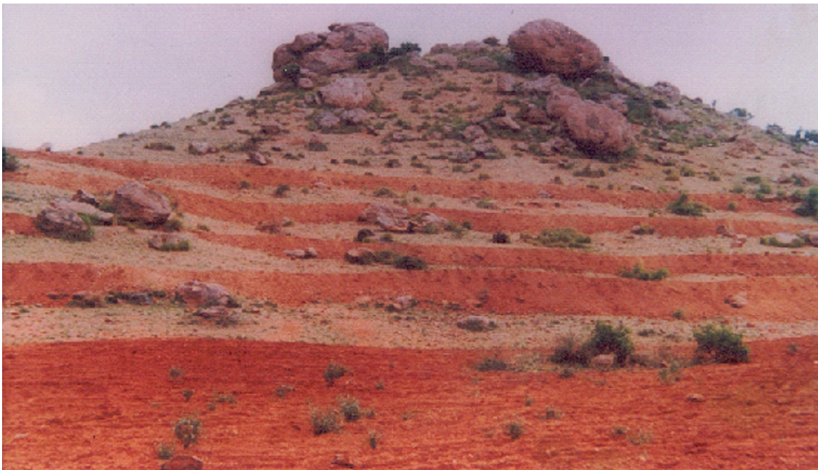
Fig. 14. 9 Continuous contour trenching
