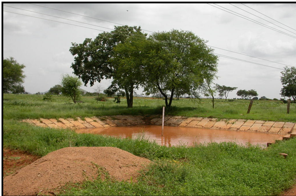
Fig. 15.2 Farm Pond Lined with Kadapa Slabs
