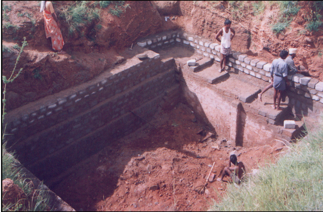
Fig .15.3 Farm Pond lined with Cement Bricks
