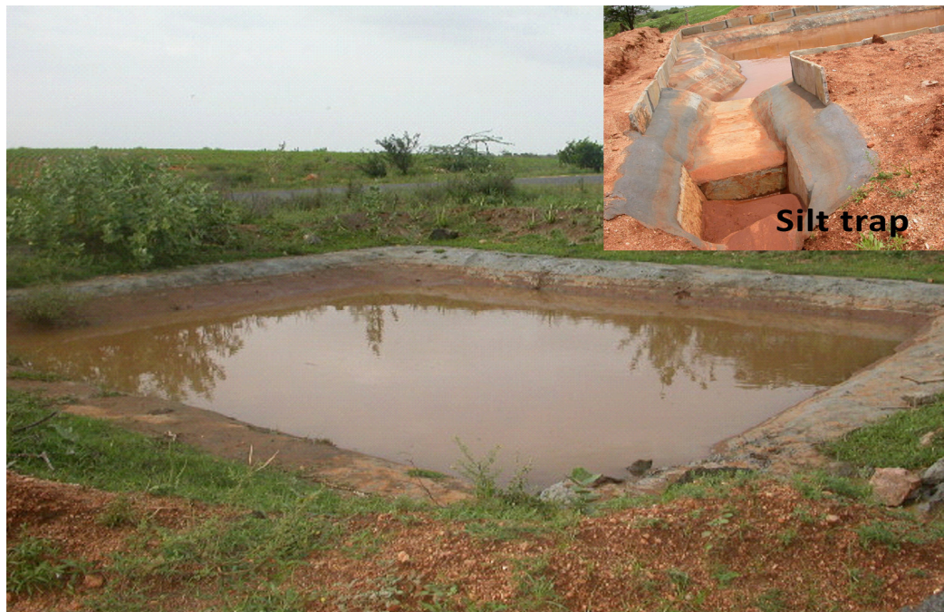
Fig: 15.5 Farm Pond lined with soil + cement (6:1 ratio)
