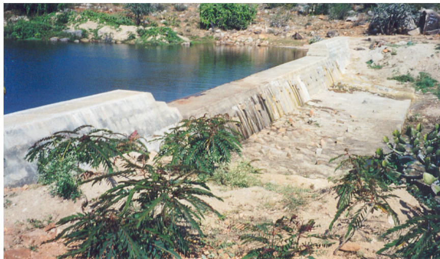
Fig. 14.6 Concrete check dam for gully control
