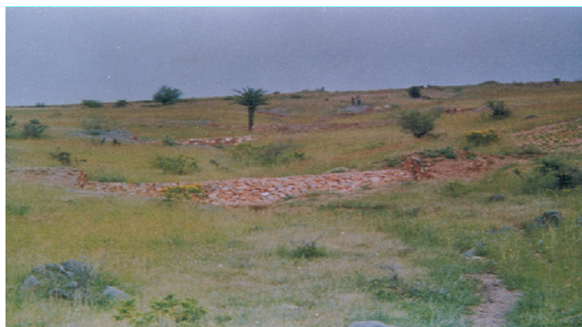
Fig. 14.7 Loose boulder check dam for gully erosion control
