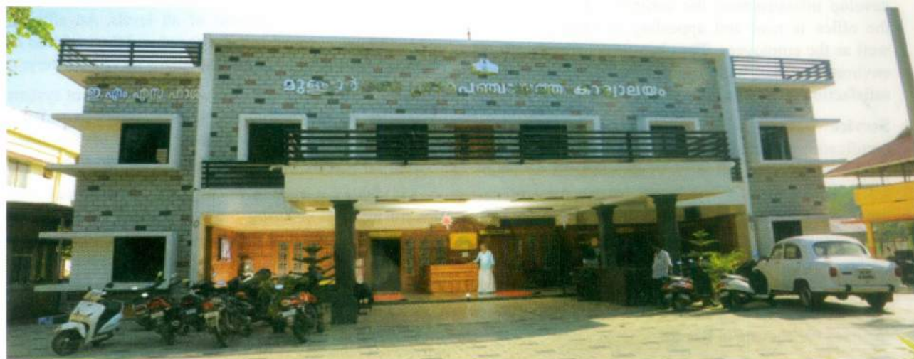
Mullurkara Gram Panchayat Office in Thrissur District, Kerala
