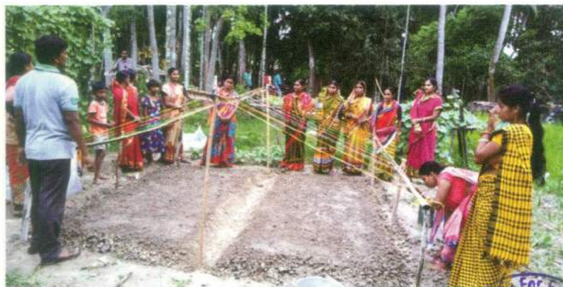
Handholding Training on Construction of Rainshelter
