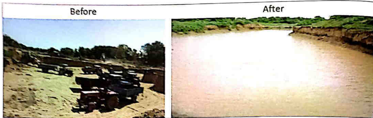
Figure 9: Before after images of water conservation work in Ranej village. Banaskantha. Increase in storage capacity by 5 lakh cubic feet.
