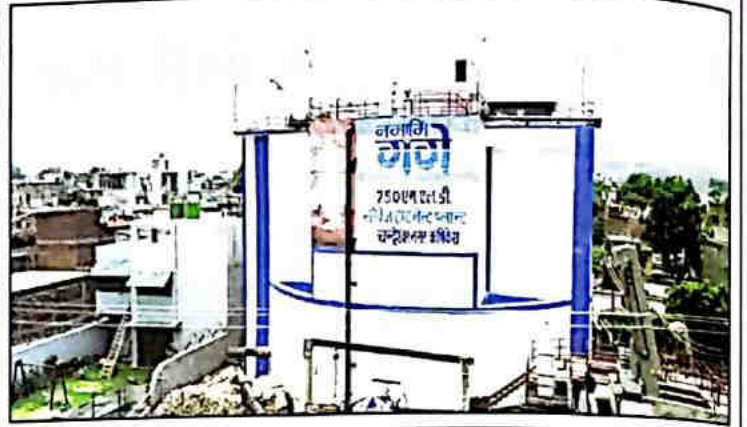
7.5 MLD STP, Chandreshwar Nagar, First four storey STP
