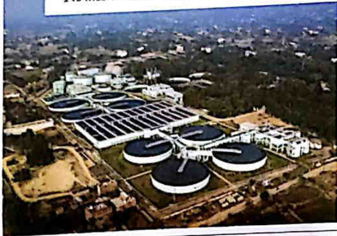
140 MLD State of the Art STP at Dinapur, Varanasi
